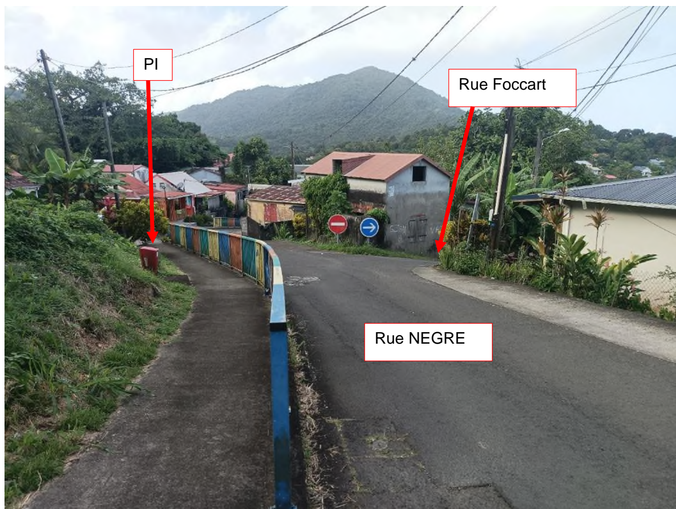
Figure 25 : Poteau incendie existant
